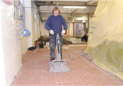
Vibrating the tiles into the cement slurry
