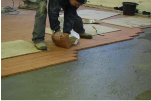
Laying the tiles
