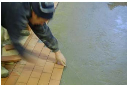
Laying the tiles
