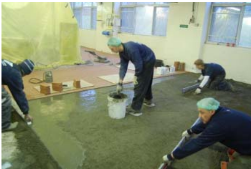
Laying the cement slurry
