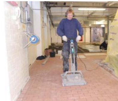
Vibrating the tiles into the cement slurry
