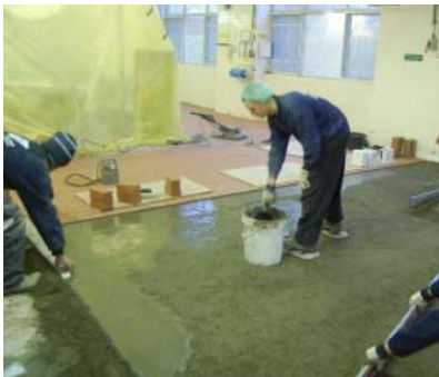
Laying the cement slurry
