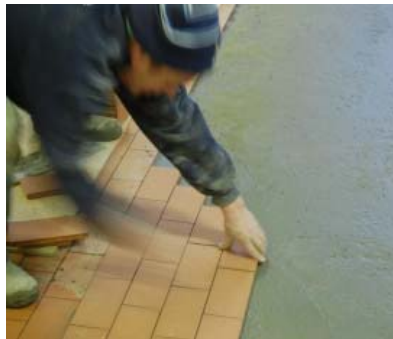
Laying the tiles
